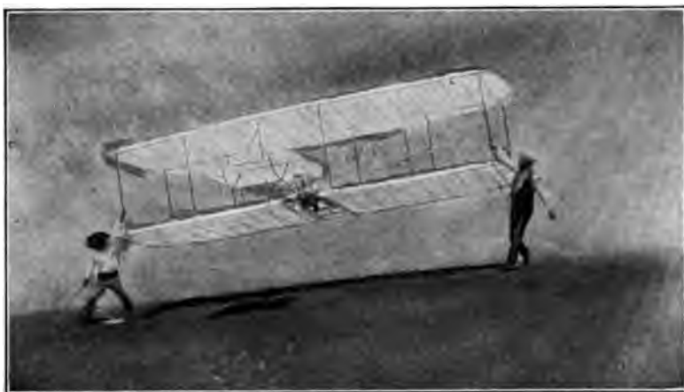
Fig. 6. Testing the Balance of a Glider with a Man Aboard
